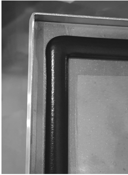
Polyurethane poured-in-place door gasket
